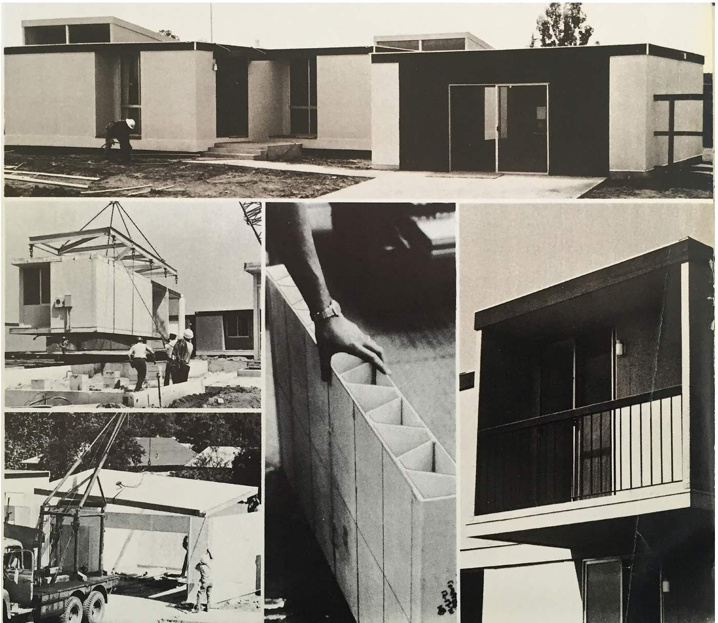
Figure 3: Material Systems Corporation houses, assemblies, and materials for Operation Breakthrough. 1972. (source: United States, Department of Housing and Urban Development, Operation Breakthrough (Washington: U.S. Dept. of Housing and Urban Development, 1972) 20.)
